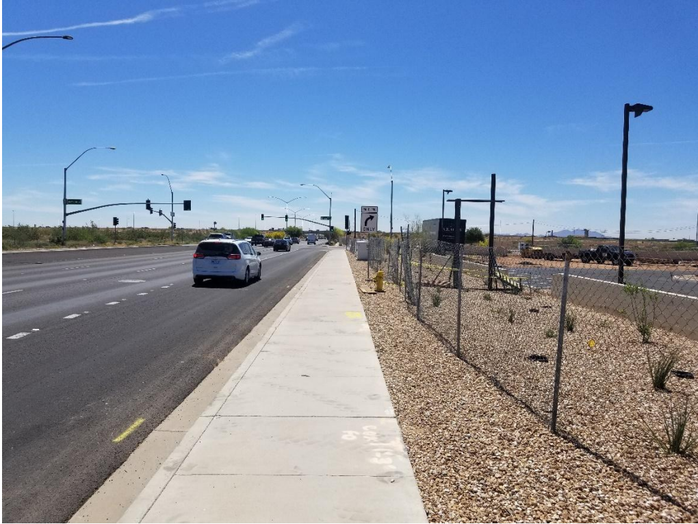
NE Property Corner Looking South
