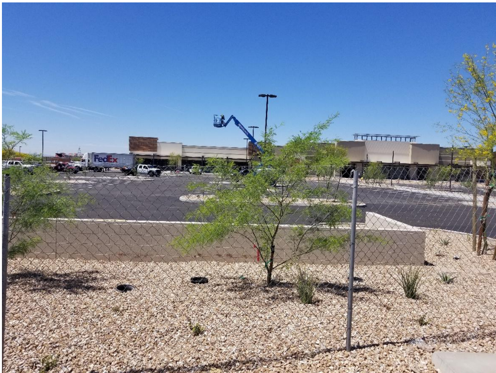
NE Property Corner Looking West
